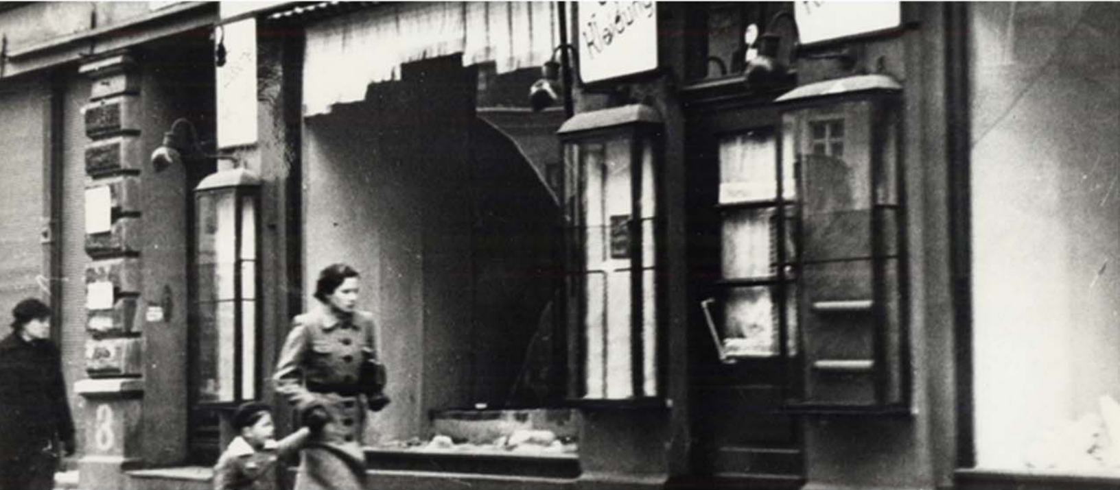
This photograph shows a Jewish shop destroyed during the pogrom of Kristallnacht. This picture was taken on November 11th in Magdeburg, Germany.
